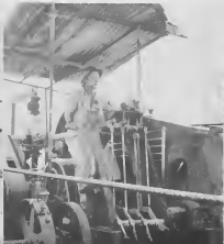
MANNING THE guyed derrick's hoist is W. Wernot, operator from Mechanical-Garage (Transportation). The steam powered hoist has three drums. OPERANDO E hoist di e derrick ta W. Wernot, operator di Mechanical-Garage (Transportation). E hoist cu ta move cu steam tin dres drum.
